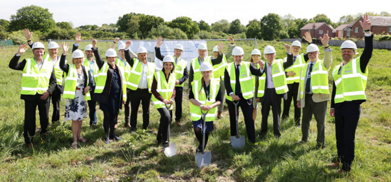
Breaking ground: We celebrate the start of work on the £13.5million centre in May 2022.
